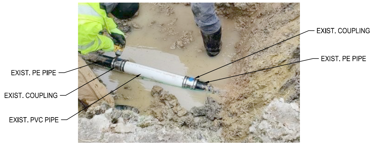
PHOTO: EXISTING CONDITONS
