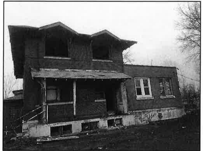
Side view of the “Mansion” office building prior to demolition (March 2021).
