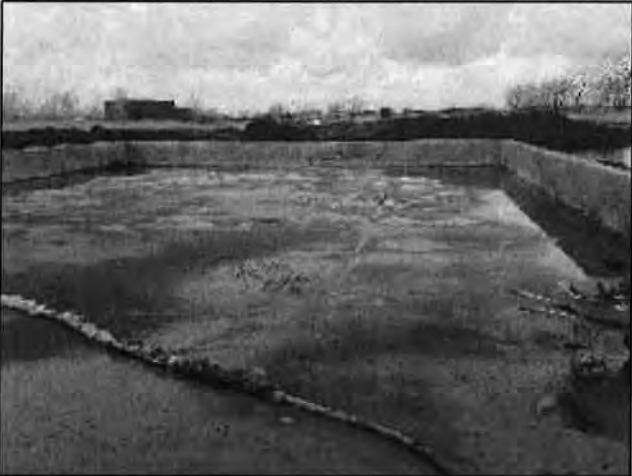
Top: Mixing Pad prior to cleaning (September 2020) Bottom: Mixing Pad post cleaning of tar and coal residuals (April 2021).
