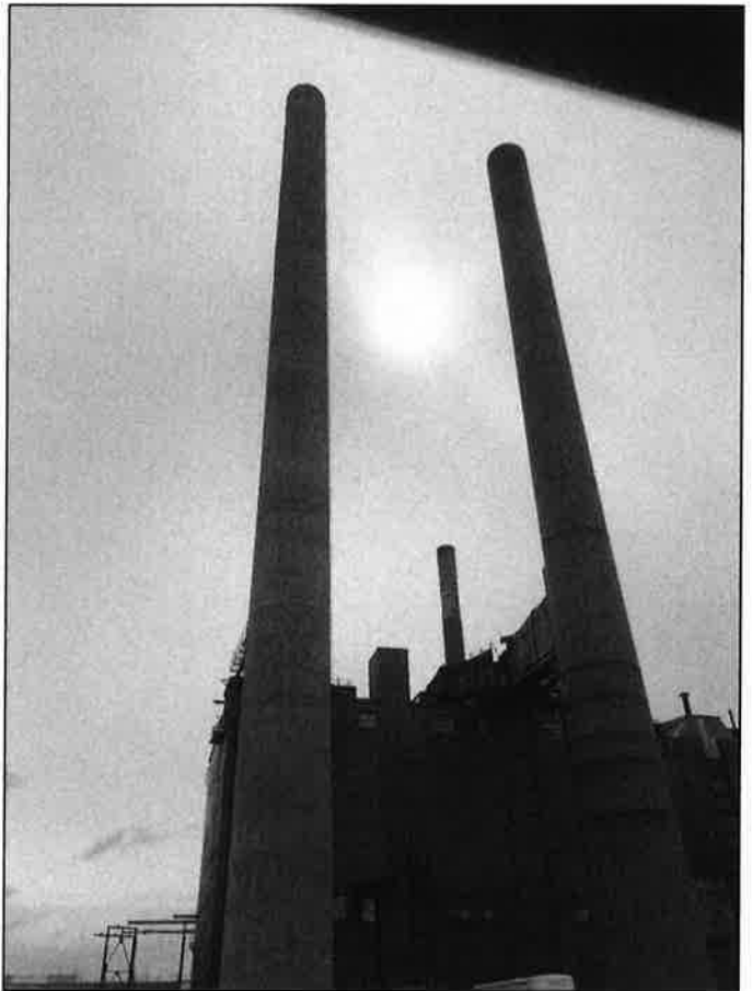
The two boiler house stacks (forefront) and the top of the waste heat stack (center-back), looking south. All three stacks will be demolished during Summer 2021 (March 2021).
