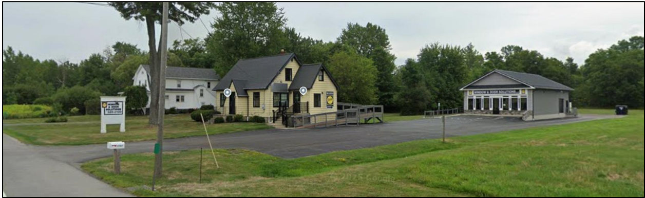
7767 Transit Road – Street View
