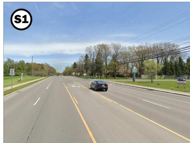
SPUR #1 SHERIDAN DR. & EASTERN HILLS MALL DR. Sheridan Dr. looking east towards the point of intersection with the Eastern Hills Mall access drive.
