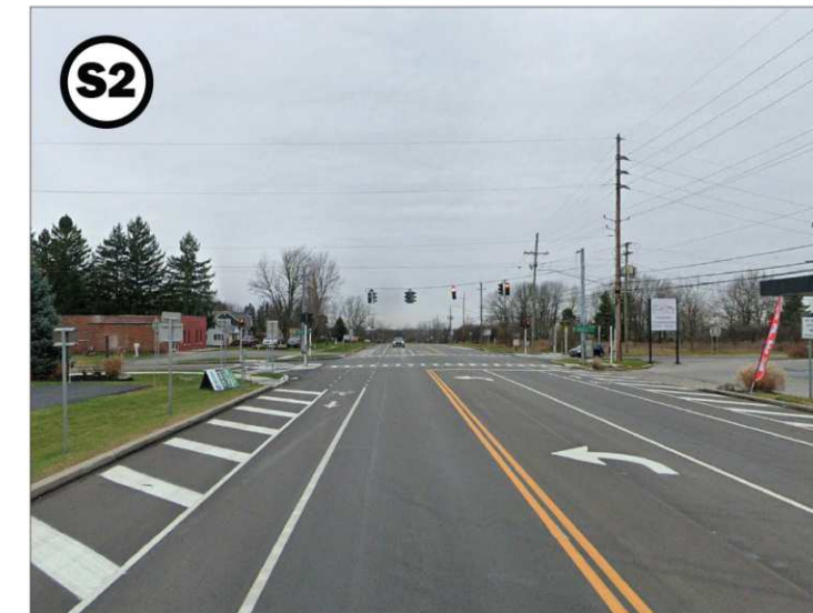
SPUR #2 SHERIDAN DR. & SHIMERVILLE RD. Sheridan Dr. looking west towards Shimerville Rd. intersection.
