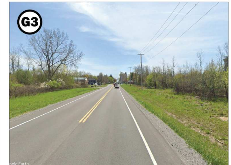
CORE GATEWAY #3 HARRIS HILL RD. SOUTH TO SHERIDAN DR. Harris Hill Road looking south towards the point of intersection with Sheridan Drive (where double yellow line begins).
