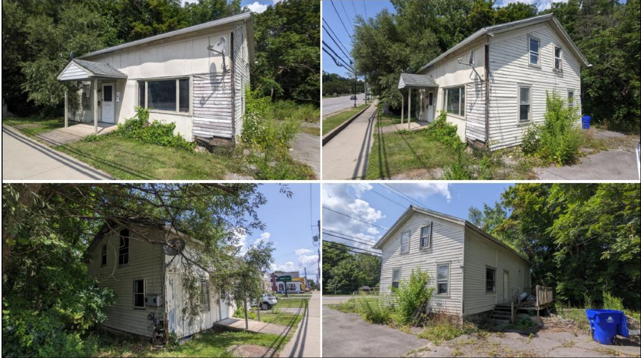
10594 Main Street Demolition Info
