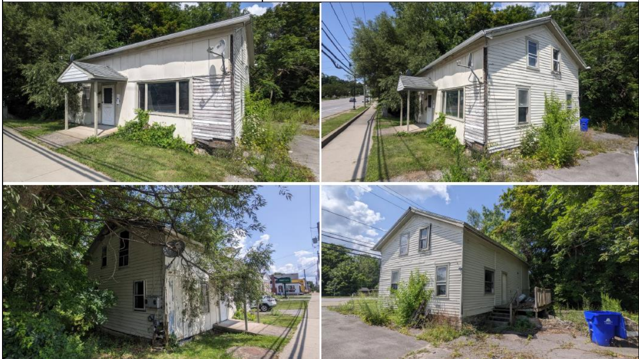
10594 Main Street Demolition Info
