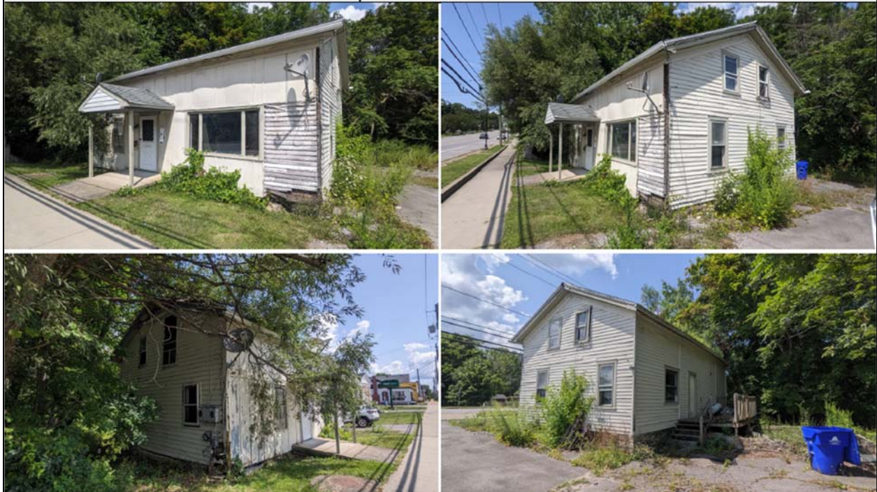
10594 Main Street Demolition Info
