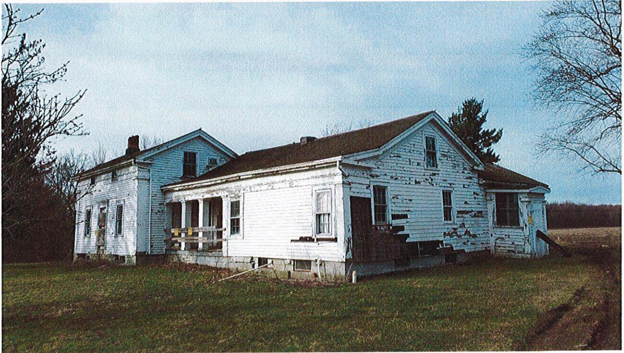
Photo 1. Overall view of house facing northeast corner.
