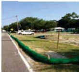
Definition & Scope A temporary sediment control practice composed of a degradable permeable mesh tube filled with compost filter socks to filter sediment and other pollutants associated with construction activity to prevent their migration off-site.
