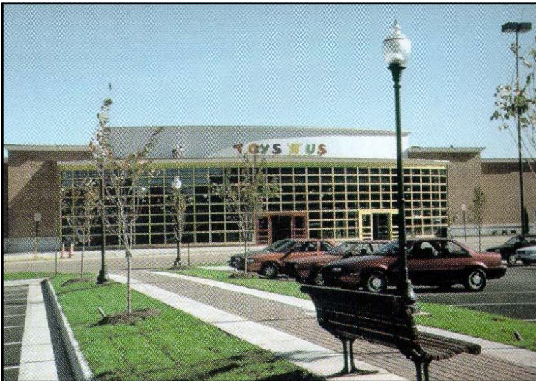
Figure III-23: Example of pedestrian accommodations provided in large parking area
