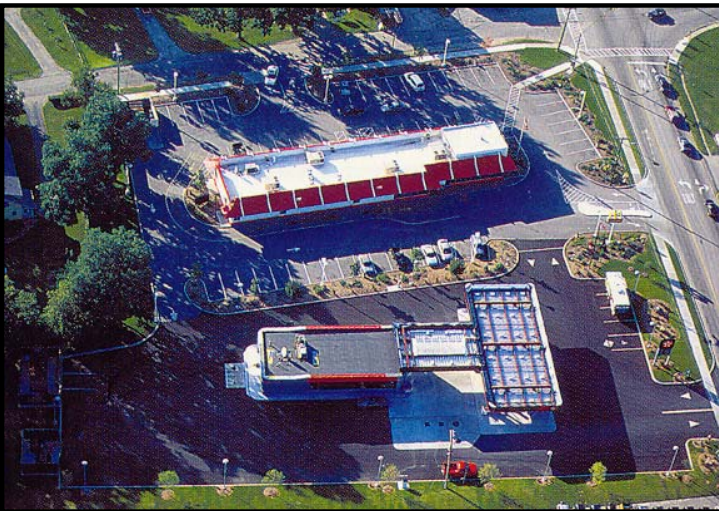
Figure I-6: Highway commercial uses that are interconnected and have access to the lower volume side road.
