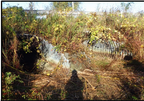
Existing Photo: East elevation of structure.
