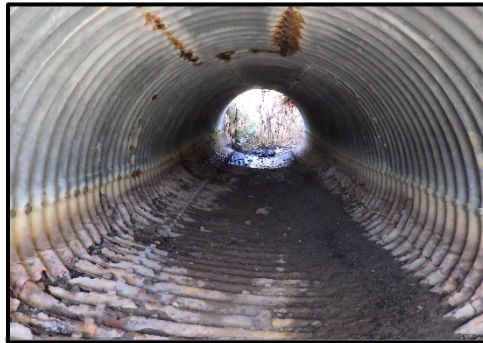
Existing Photo: Taken on the east end of the structure, looking west in Span 1.
